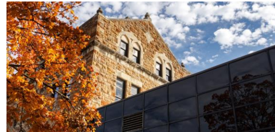
Building Renovations and Additions
